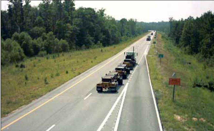
The inaugural cycle of testing began in the summer of 2000 and was basically a study of surface mix performance. The test sections were rebuilt in 2003 for the second cycle of testing then again in 2006 for the third cycle, both times with a combination of mill/inlay surface mixes and variable thickness structural sections at the discretion of each participating state.
