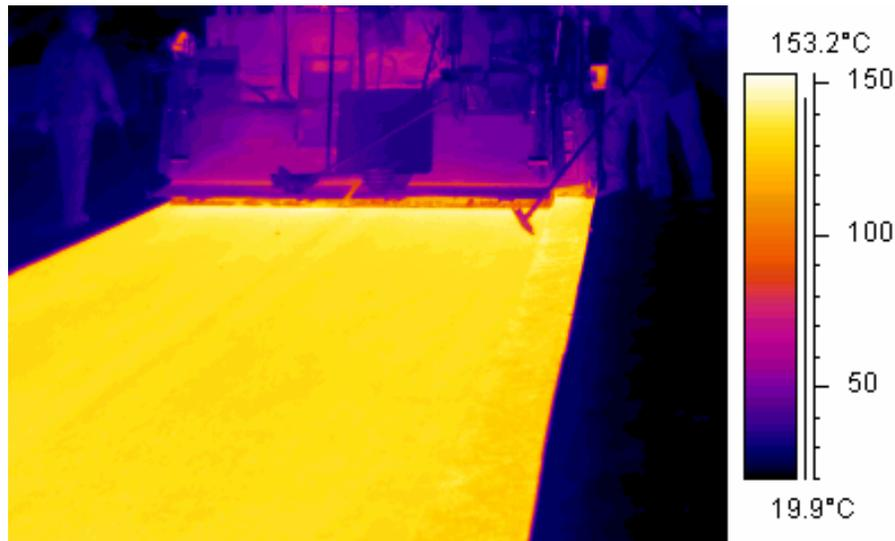
Figure 5: Thermal profile of a pavement where a MTV was utilized.
